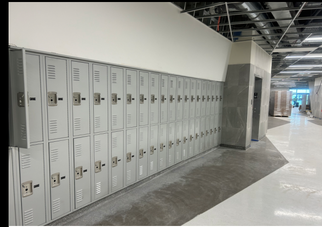
Lockers and Corridor Wall Tile
