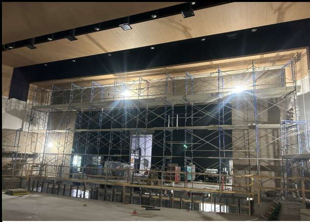
Brick Façade at Auditorium Stage
