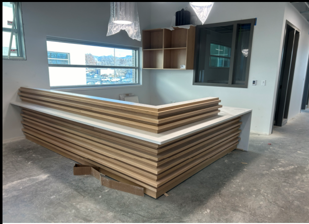
Casework at Front Office
